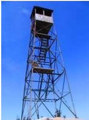
Hurricane Mountain fire tower (Source: Wikipedia) (click image to enlarge)
