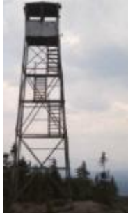
St. Regis fire tower (Source: Friends of St. Regis)
